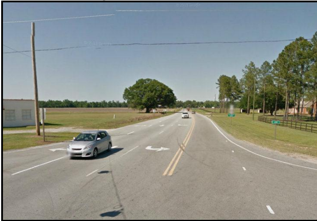
Google Maps (May 2012) – Looking North US 13 - 258 Approach
